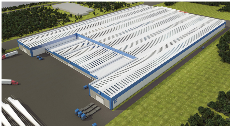
The new TPI factory in Menemen, expected to be ready in 2nd half of 2016
