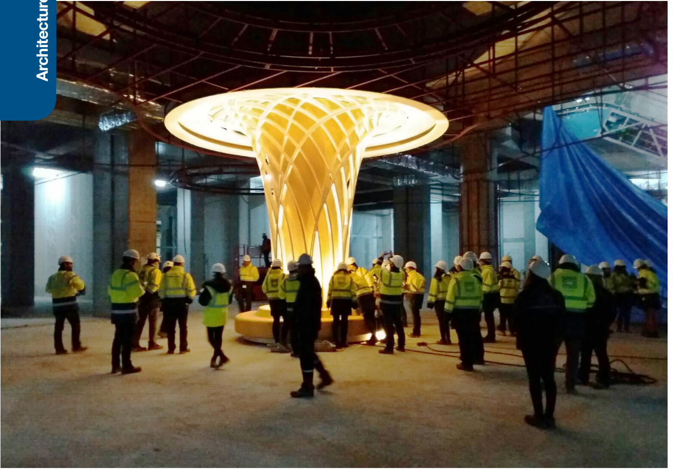
The first column installation on site for EMAAR being checked by engineers
