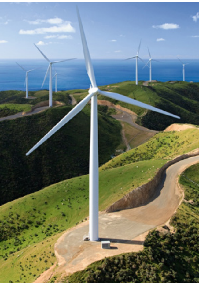
A new wind farm in Turkey
